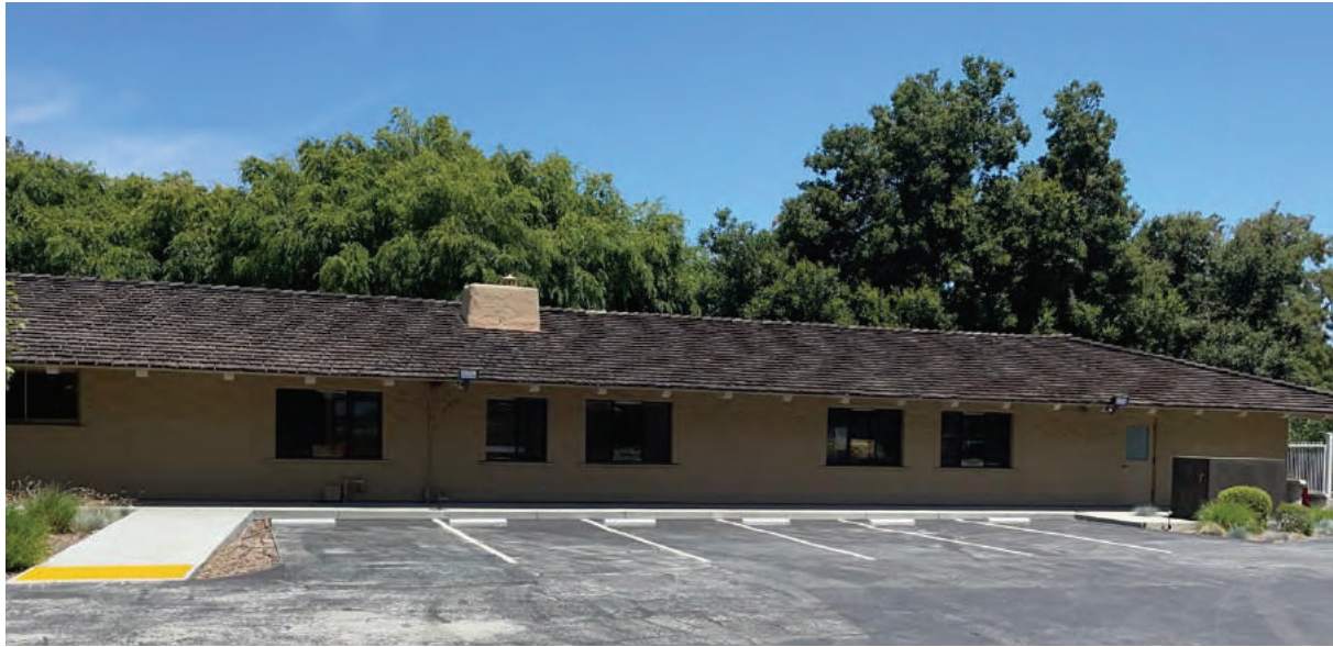
Rear elevation of east wing, interior parking lot
