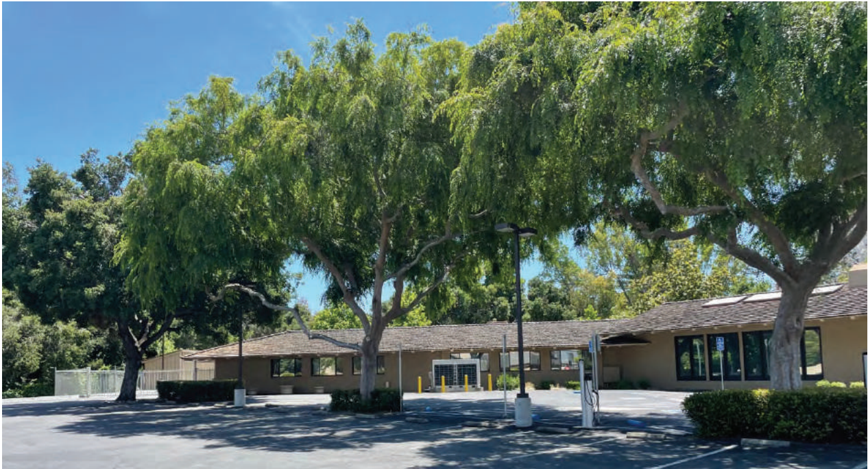
North elevation along Middlefield Road
