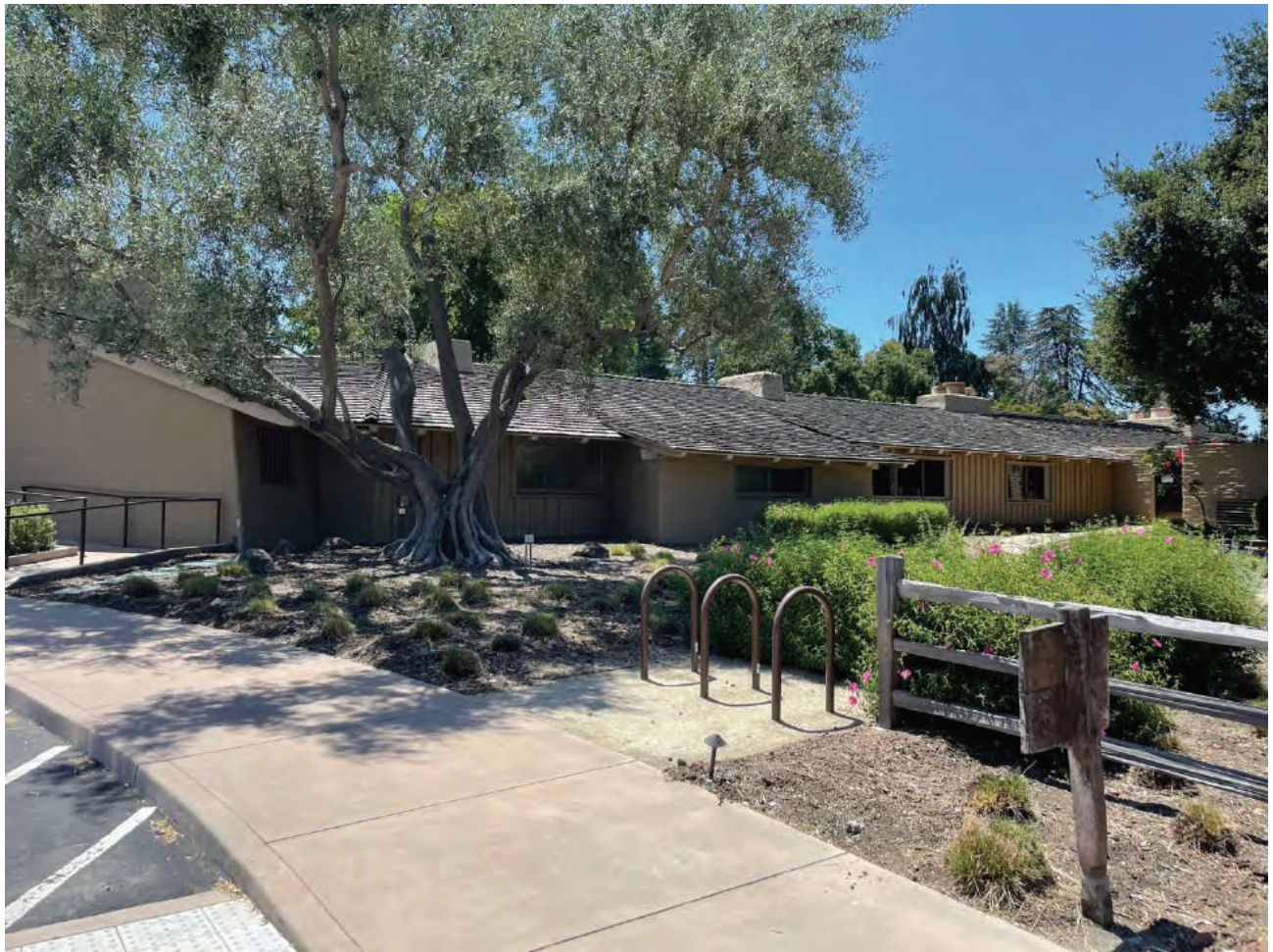
West façade of southwest wing facing Willow Road
