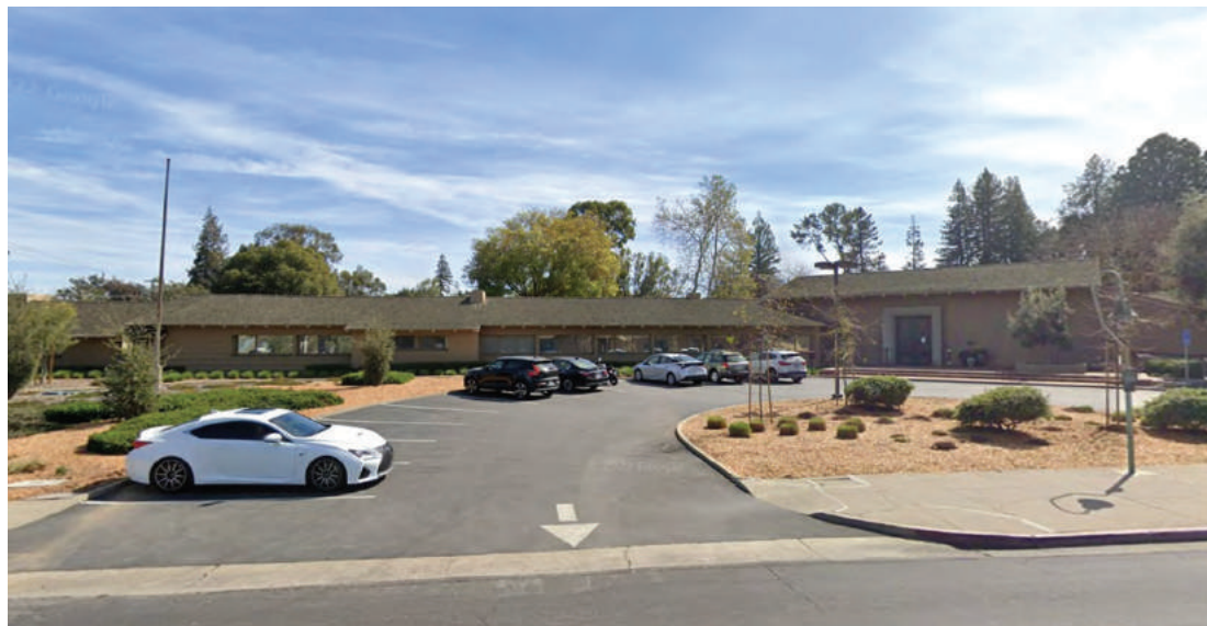
Street view of primary (west) facade
