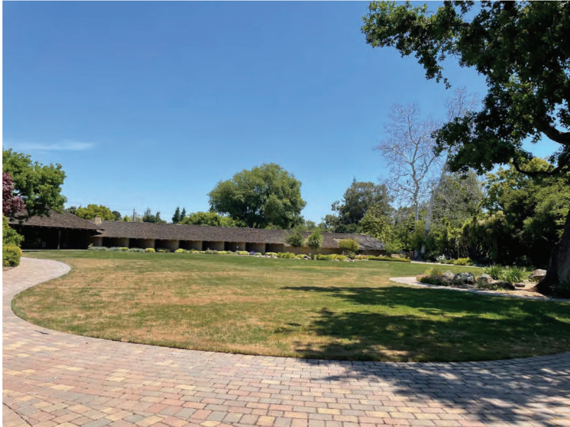
Rear (south) elevation from San Frisquito Creek
