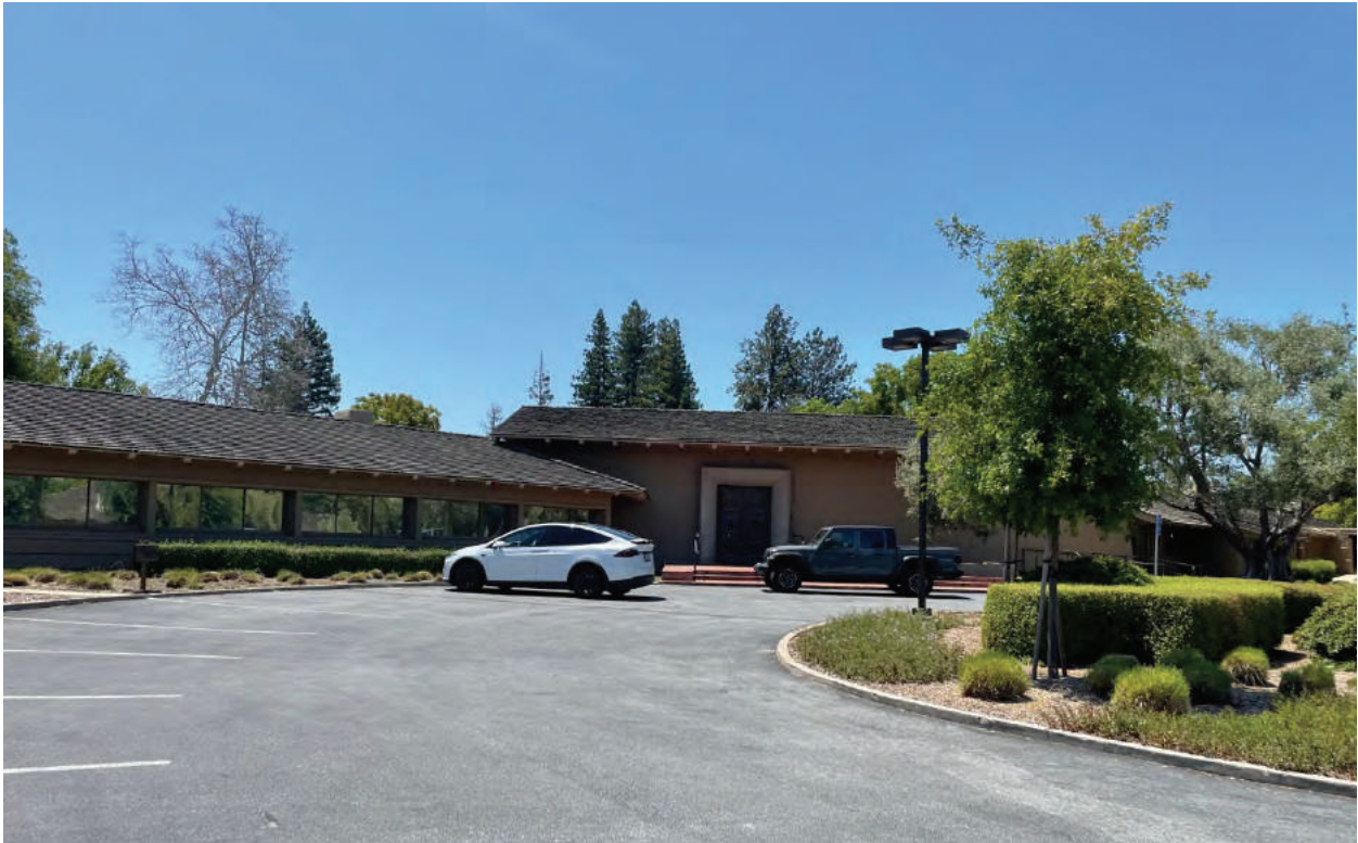
Primary entrance, main (west) facade
